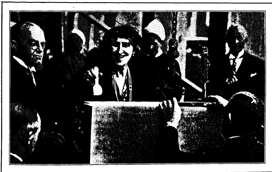
HER GRACE LADY KINNAIRD LAYING THE FOUNDATION STONE OF THE NEW NURSES' HOME.
